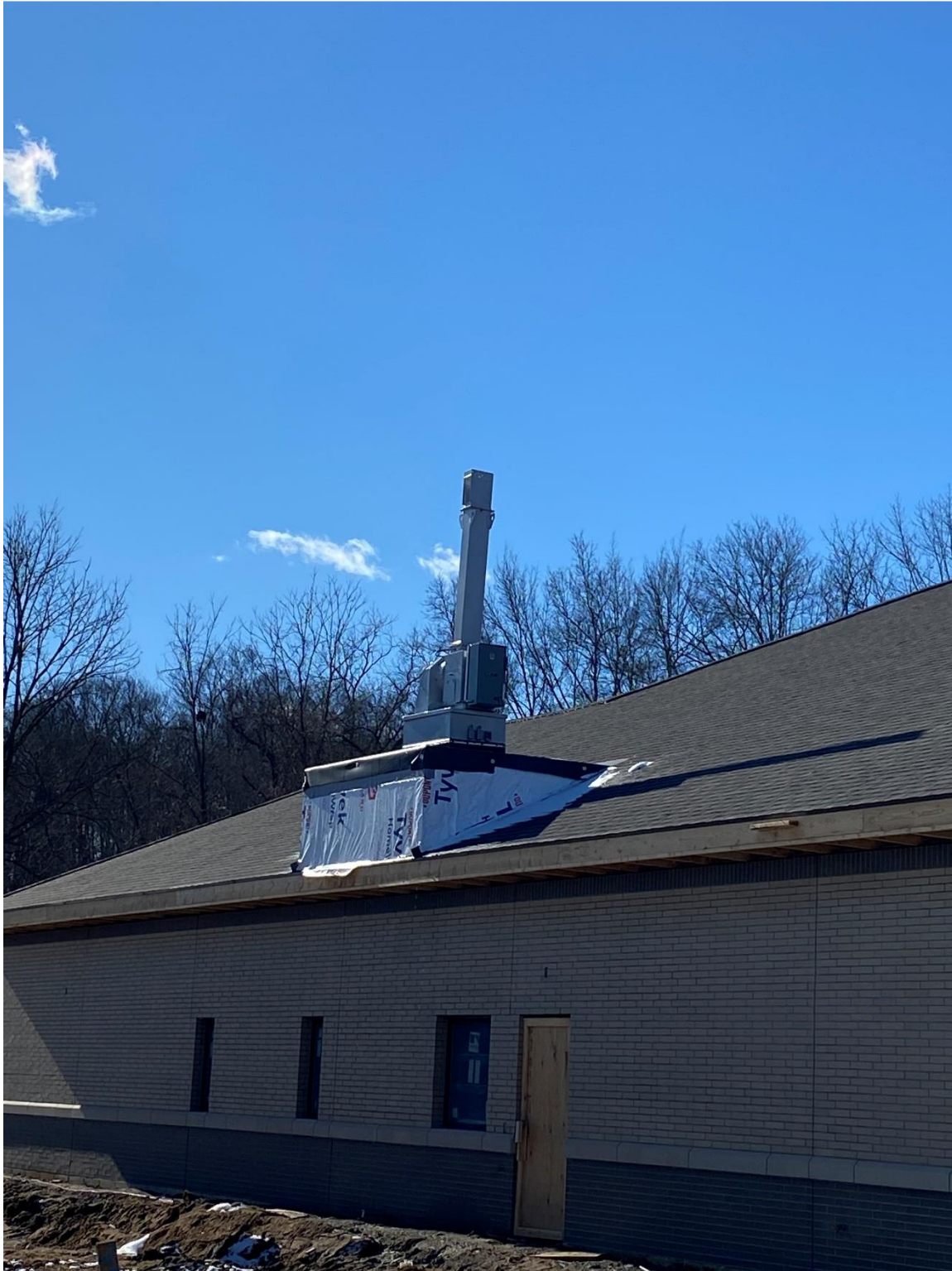
Administration Building lab hood exhaust system installation
