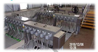
Figure 3 – Example UV Installation in a Channel
