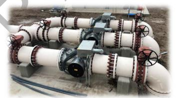
Figure 2 – Example in-pipe UV installation (Credit: Aquionics)
